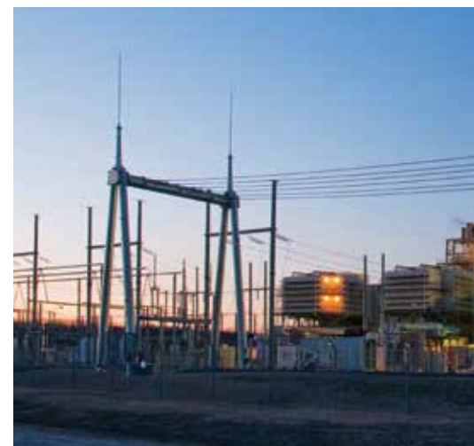
CHOUTEAU POWER PLANT
