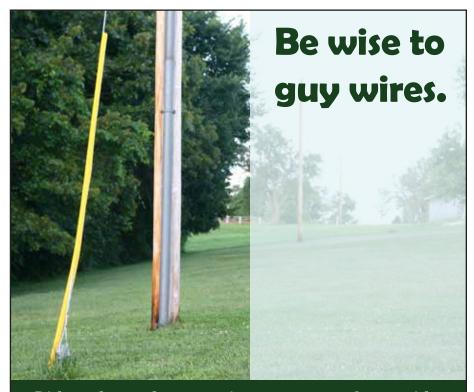
Did you know that guy wires on power poles provide grounding as well as support? Damaging a guy wire can cause an electric current disruption, creating a dangerous situation.
