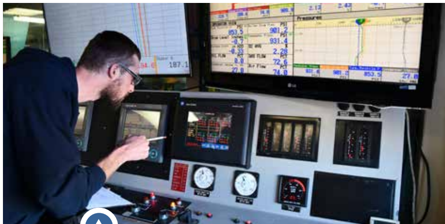
Grant Jackson, control operator, Corn Belt Power Cooperative, monitors the Wisdom Unit 1 burner control system during operation at Wisdom Station in Spencer. Wisdom Unit 1 is a 38-megawatt natural gas generating unit with fuel oil back up.
